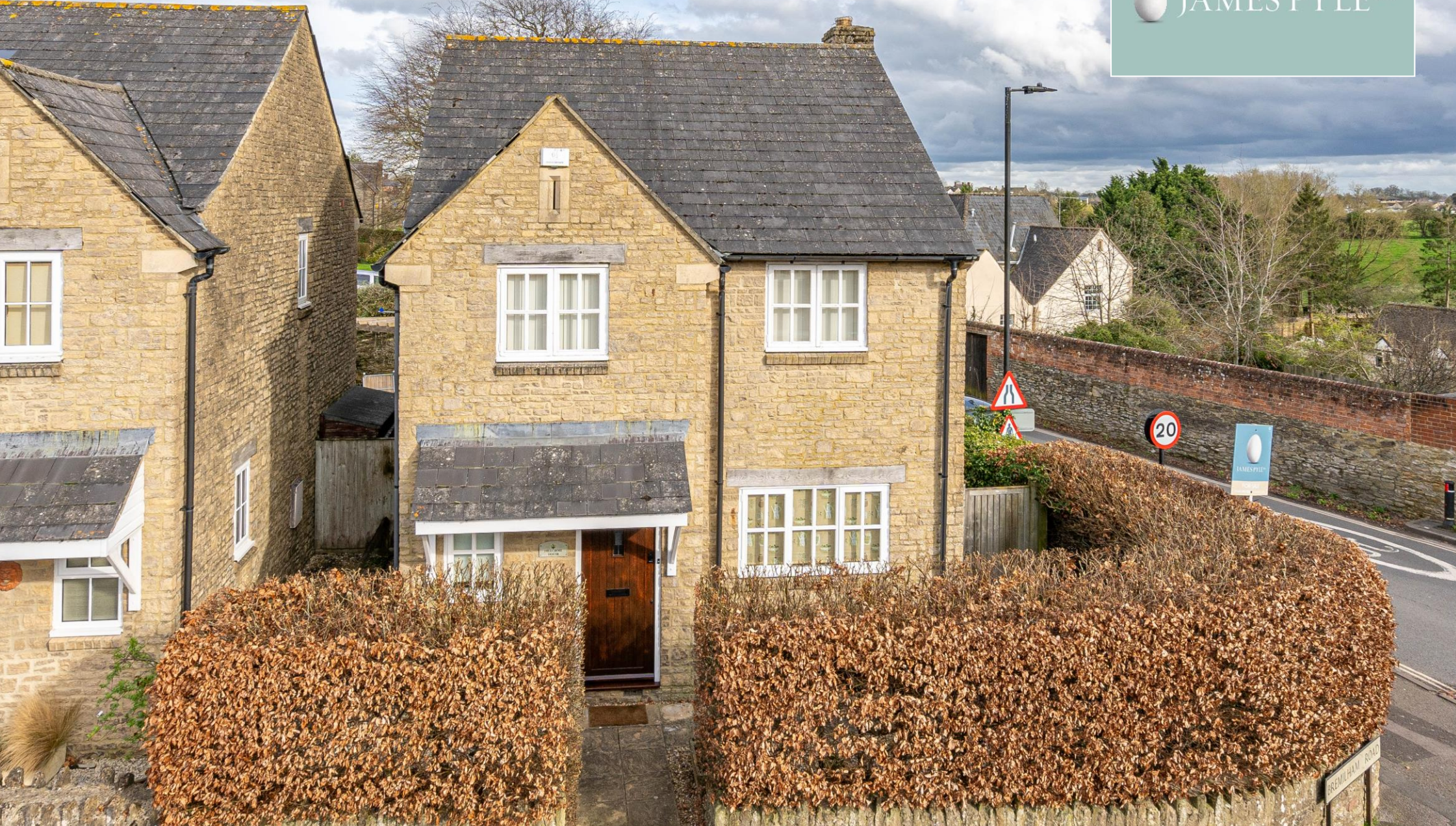
Hillcross House, 5 Holford Rise, Bremilham Road, Malmesbury, Wiltshire, SN16 0DQ
