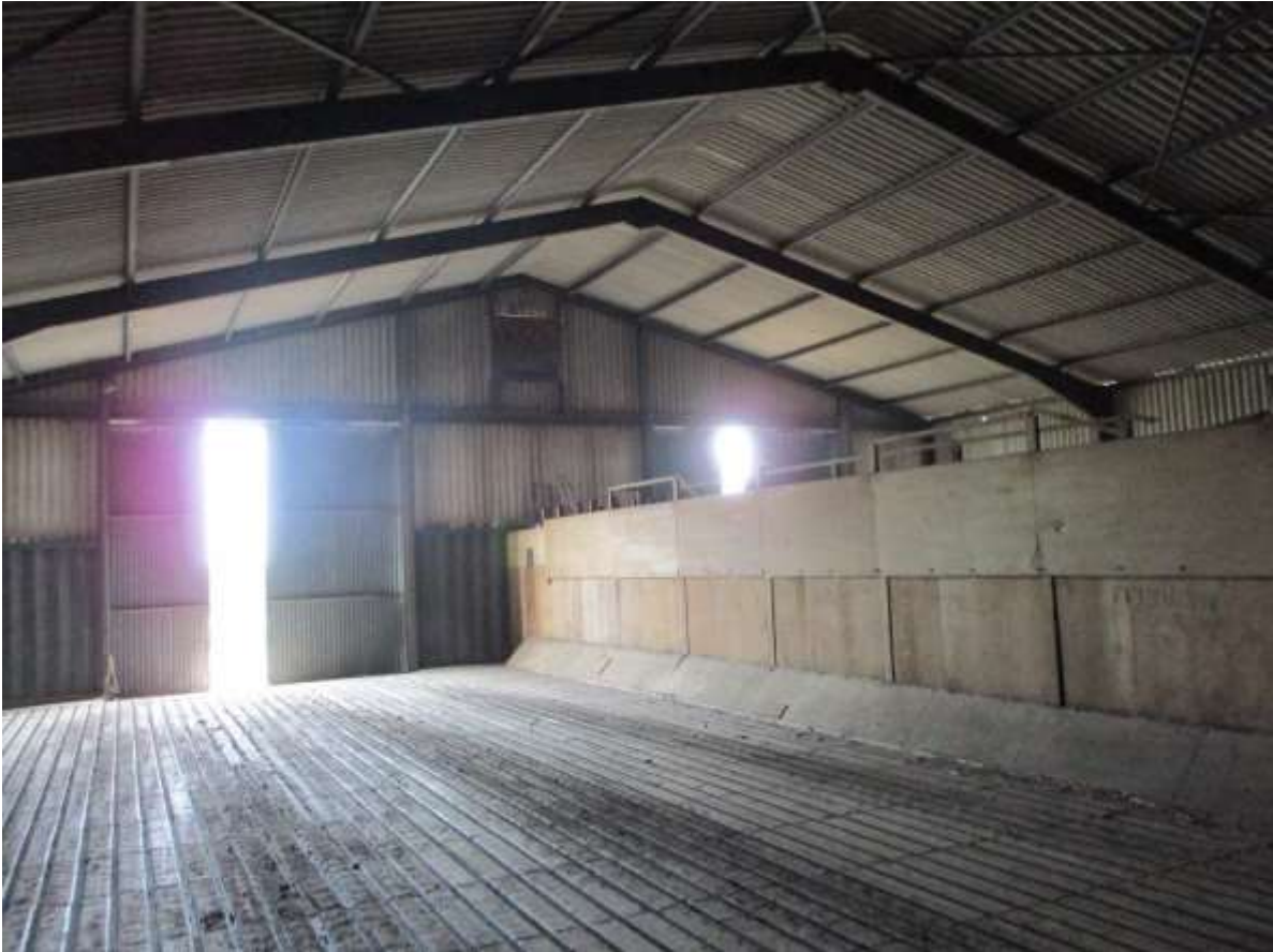
Plate 3: Internal facing main doors.
