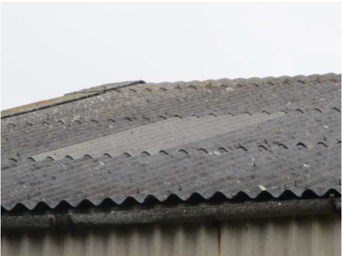
Plate 8: Previous repairs have maintained the barn in good condition.
