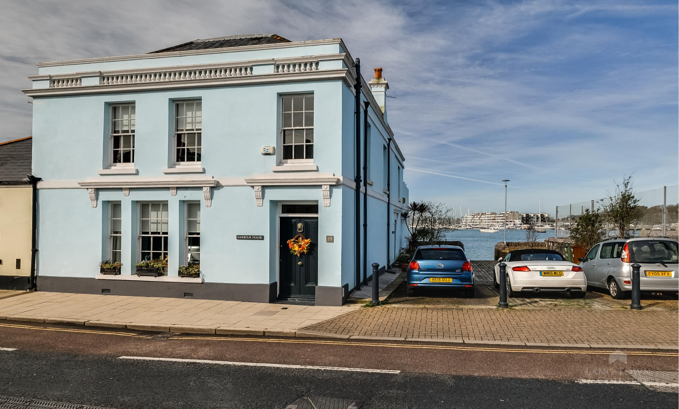
Harbour House, 19 Cremyll Street, Stonehouse, Plymouth, Devon, PL1 3RB
