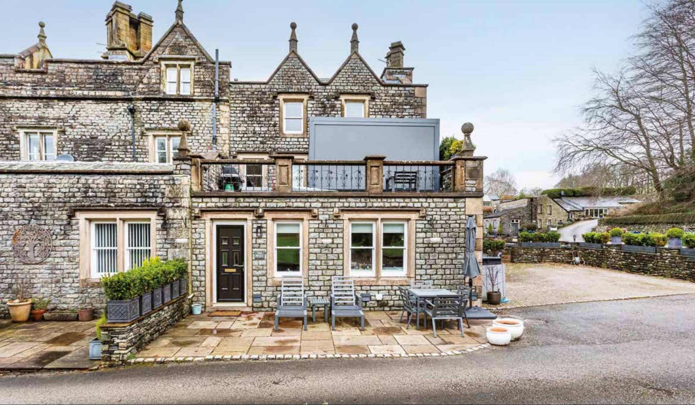
The Wing Ingmire Hall | Sedbergh | LA10 5HR
